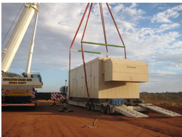
Crane operators were busy in February, March and April this year taking delivery of ten 50-tonne engine generator units at Carnarvon's new 18 megawatt (MW) Mungullah Power Station and placing them carefully on pre-laid concrete pads.
